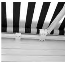
Shoulder and arm on wall mounted awning
